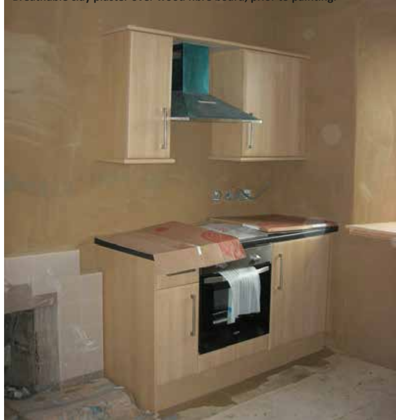
Breathable clay plaster over wood fibre board, prior to painting.
