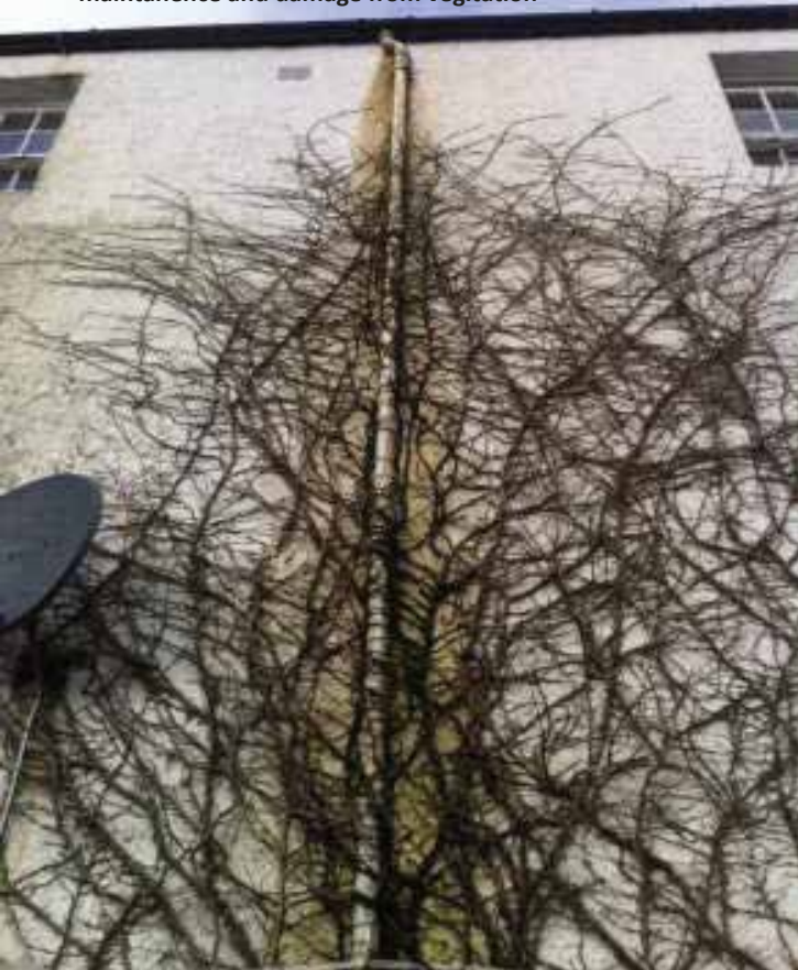
Inveraray, down pipe corroded and leaking through lack of maintenance and damage from vegetation
